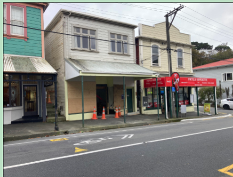
A tavern in the town? 102 Aro St still being rebuilt 29/4/25
